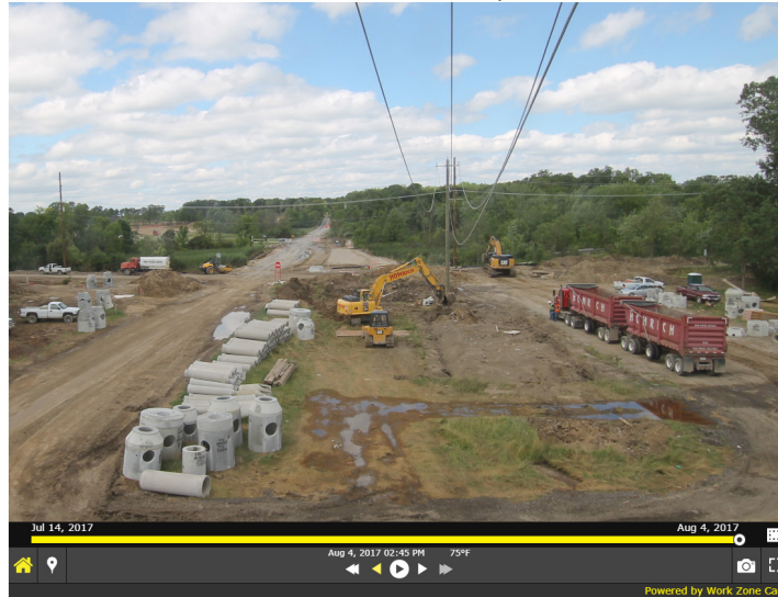
WORK ZONE CAM 10 Mile Road and Napier Road
